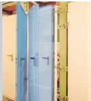
Ongoing functionality test
