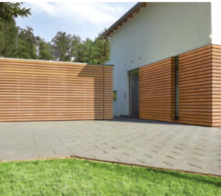
On-site cladding with timber panels
