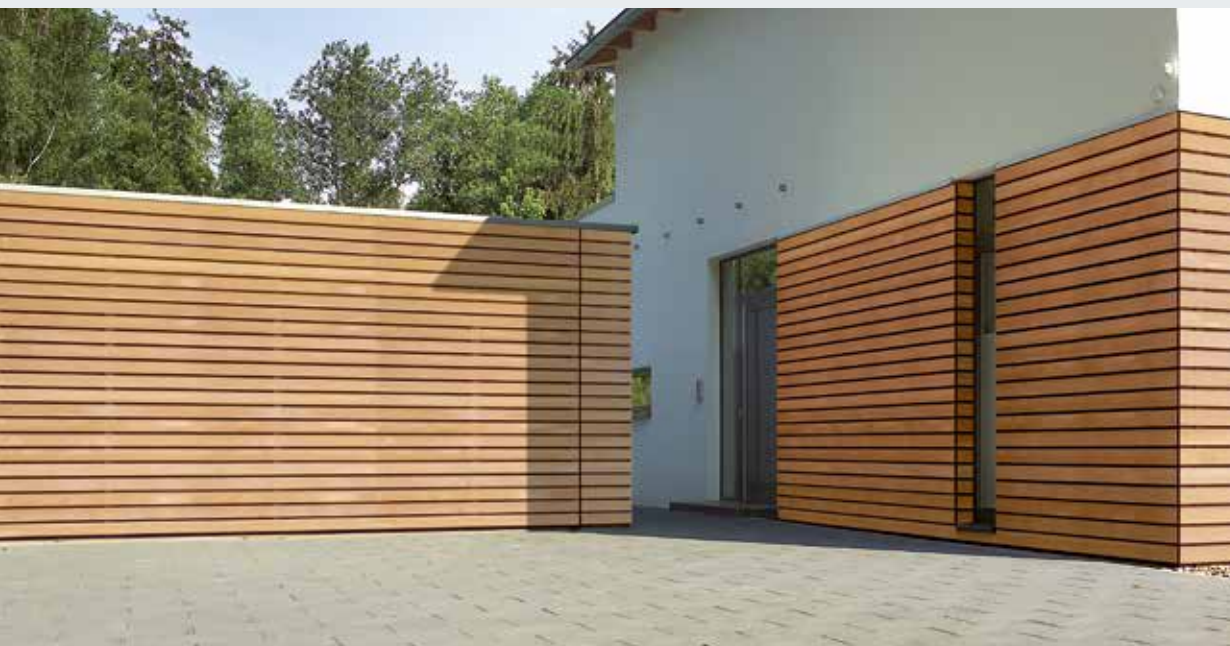
On-site cladding with timber panels
