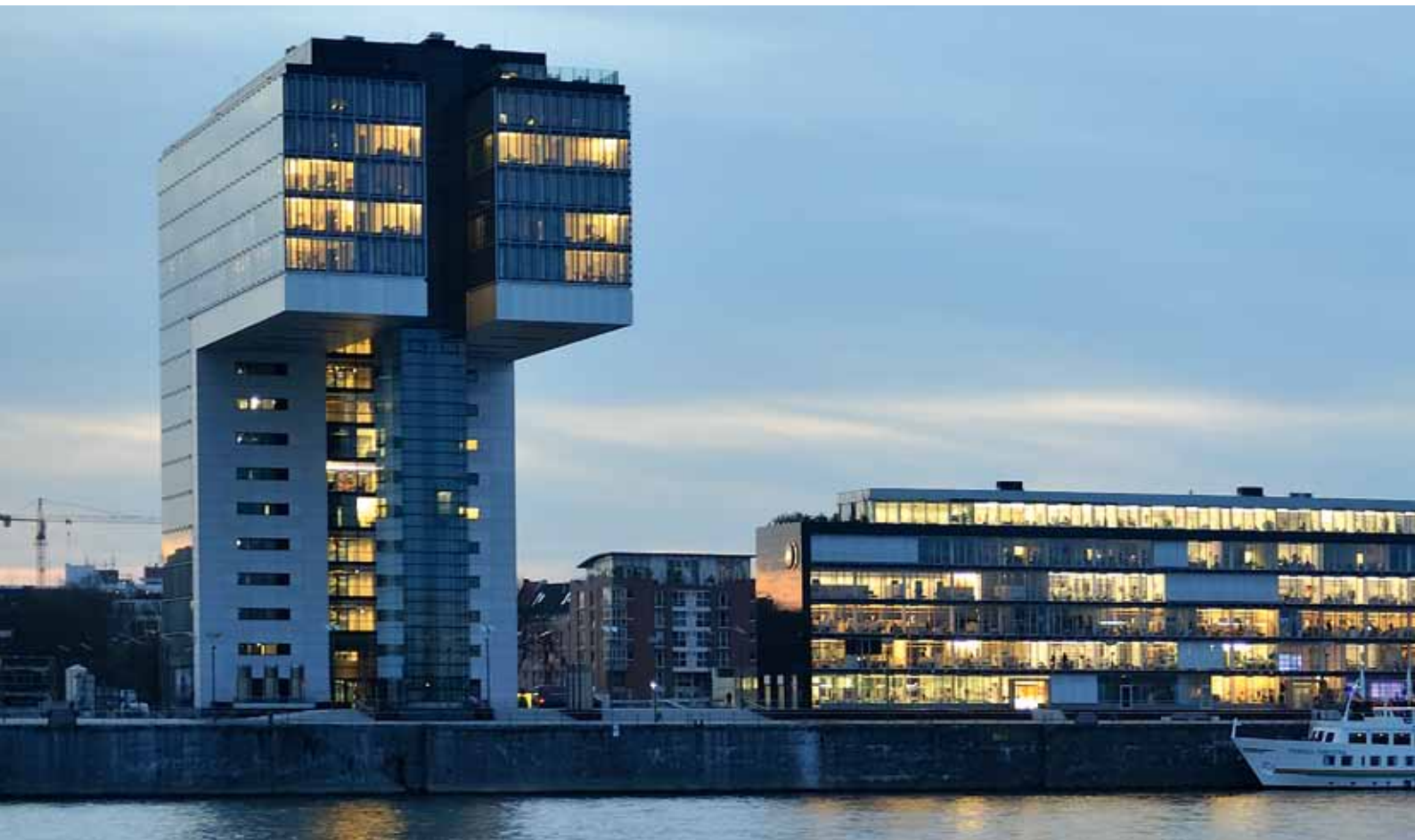
Crane buildings at Rheinauhafen in Cologne, Germany with Hörmann products
