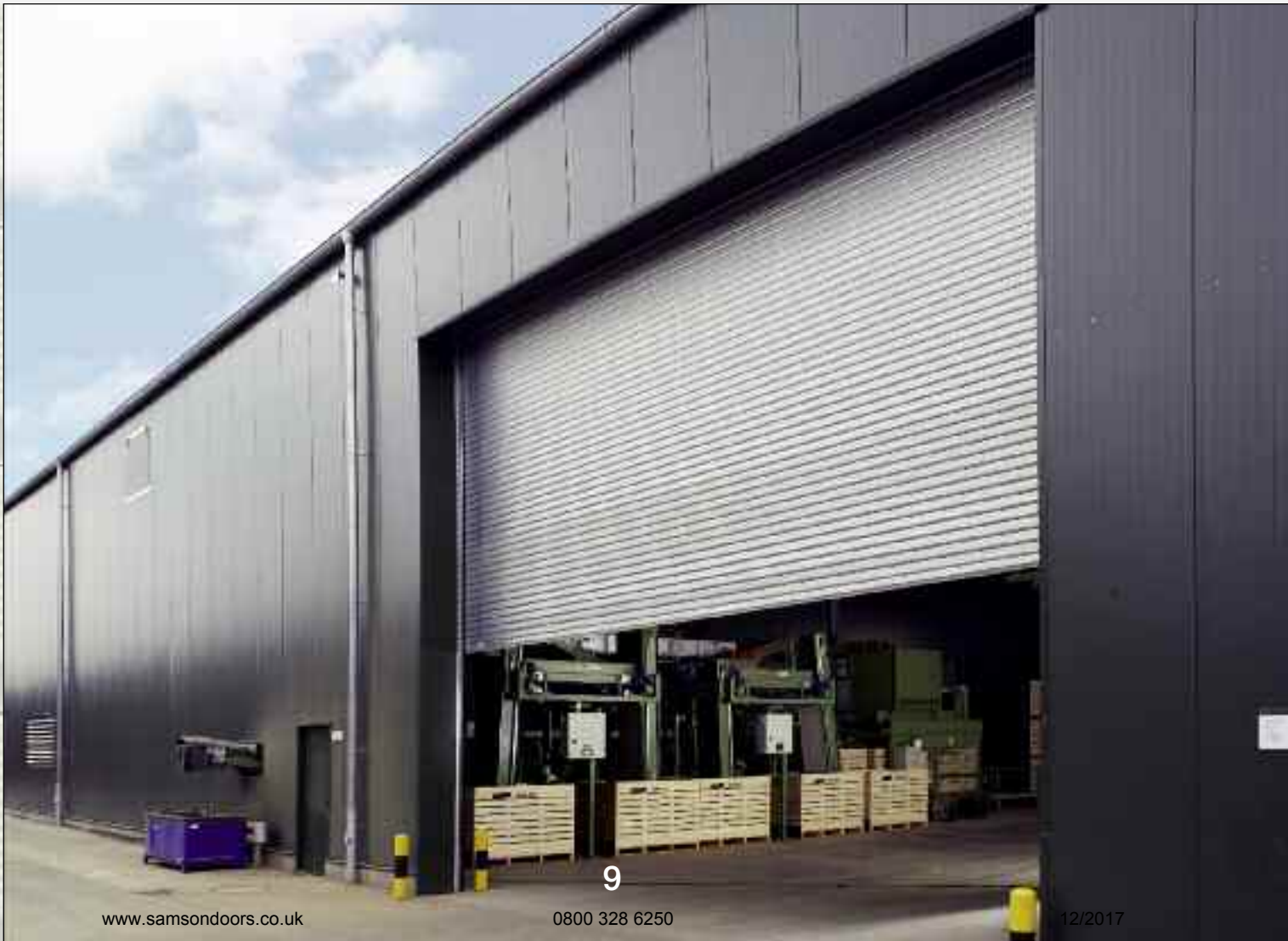
Door opening in an industrial premises.
