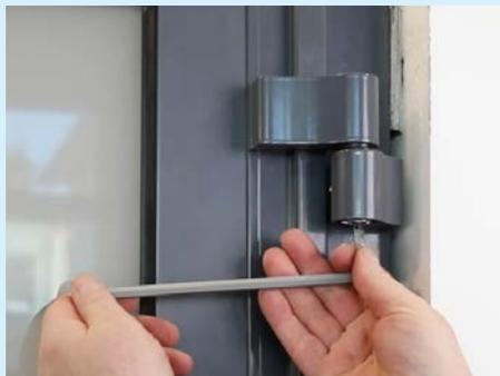
4. After adjustment, re-tighten the M6x5 set screw (4mm allen key) and refit the plug.
