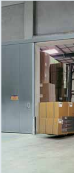
6 Fire sliding doors
