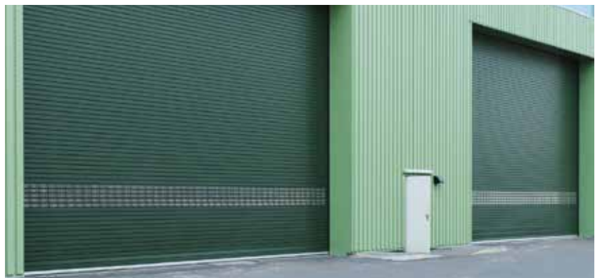
Hall closure in industrial enterprise
