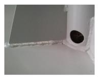
The deck plates can accommodate electrical cables. The cable that provides power to the parasol should be fed through the cable entry and protected with a suitable grommet.
