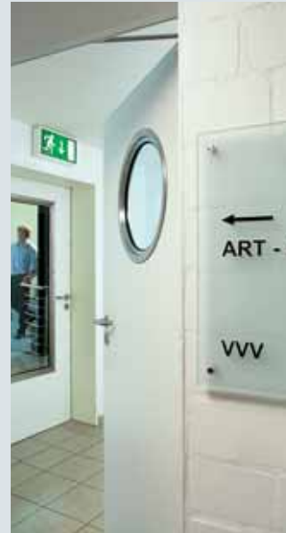
7 Multifunctional doors Facility inner doors
