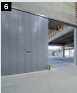
6 Fire sliding doors
