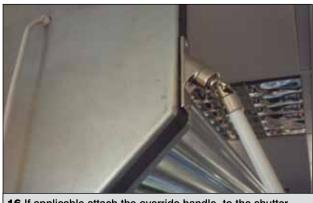
**16** If applicable attach the override handle to the shutter and test the manual override facility. Once you have identified which direction will open the shutter attach the label supplied to the override handle showing the end user which direction to wind the manual override to operate the shutter.
