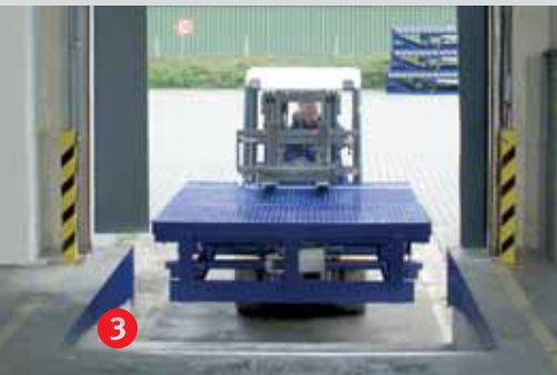
3 Insert the new dock leveller
