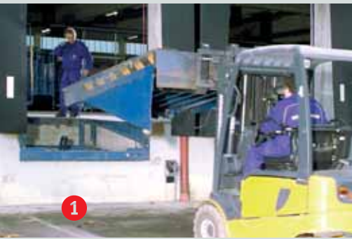
1 Dismantle and remove the old dock leveller
