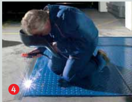
4 Weld to the edge brackets - and you're done!
