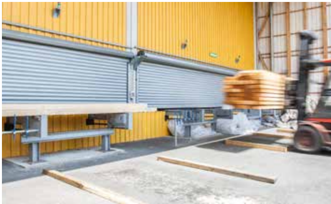
In the sawmill: Two rolling shutter doors offer sufficient room for the passage of extra wide lumber. They can also be integrated into the control systems of on-site conveyor systems.
