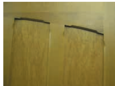
Panel detail of plywood panelled doors with cedar facings showing stopped chamfer profile
