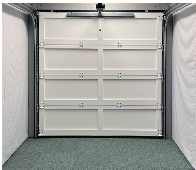
Inside view of sectional door
