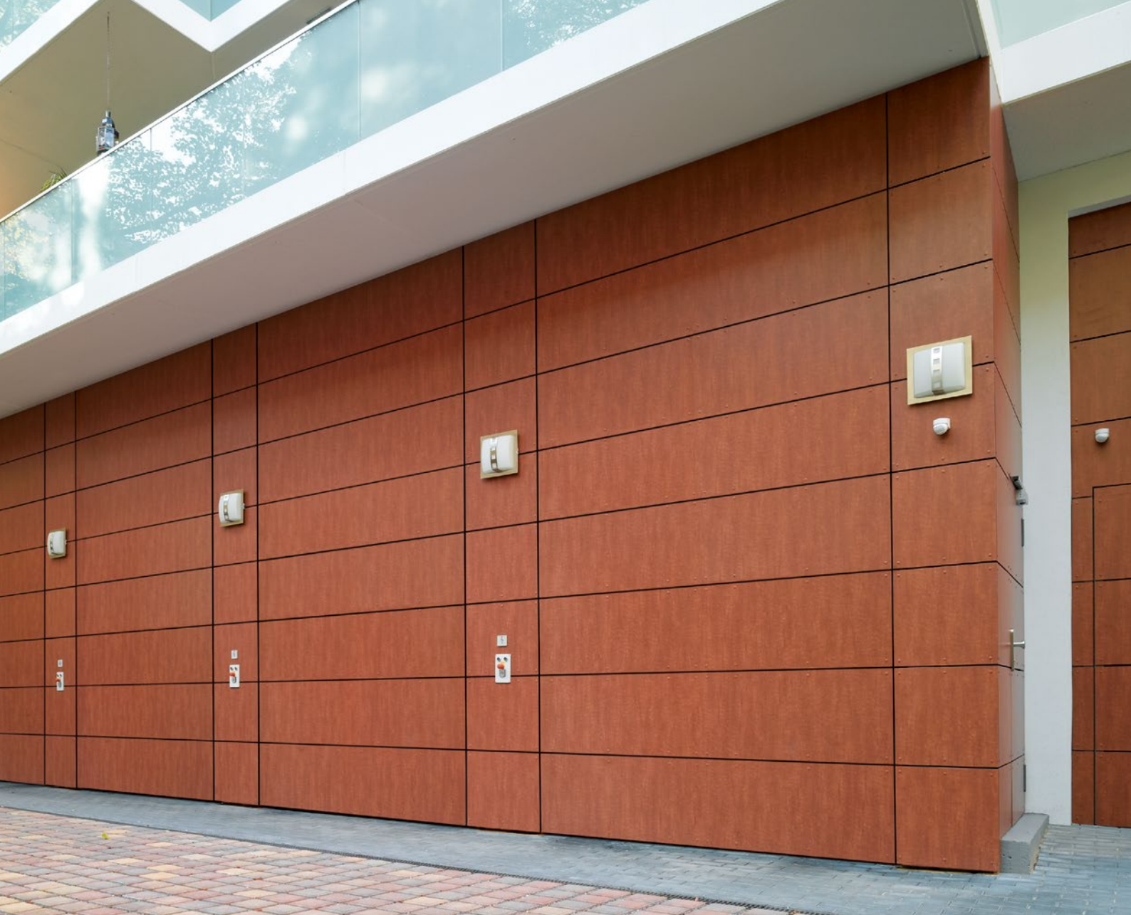
TOP RIGHT. ALR F42 with on-site flush-fitting cladding made of laminated material board
