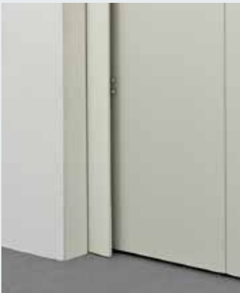
Recess flap with the door closed
