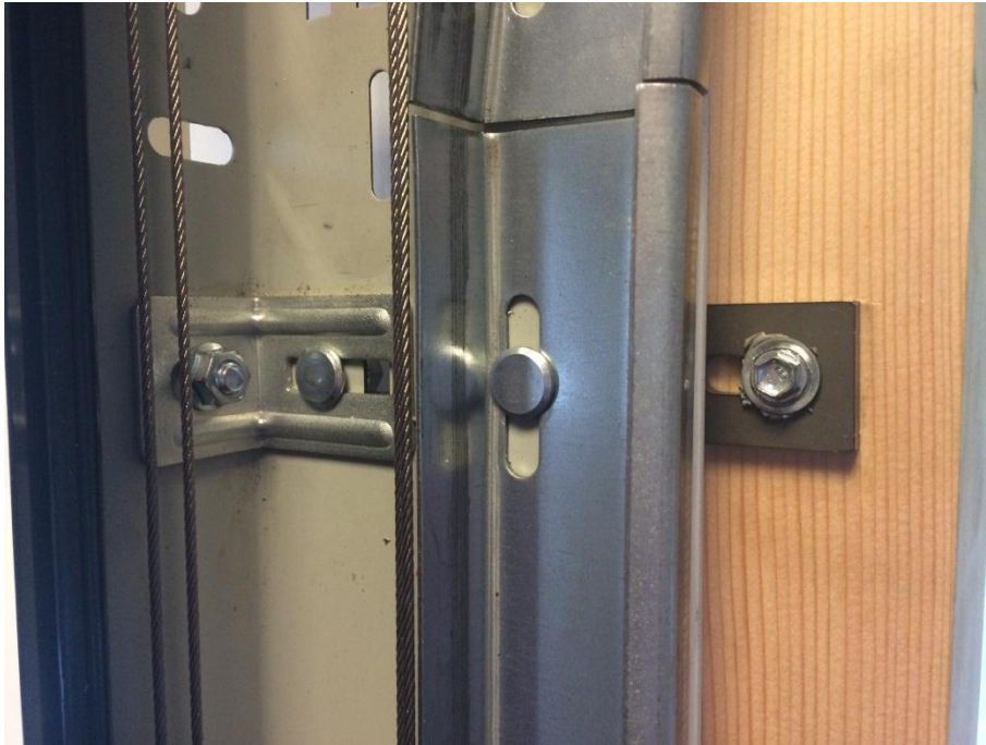
Fig 5 – Attach the bracket to your reveal
