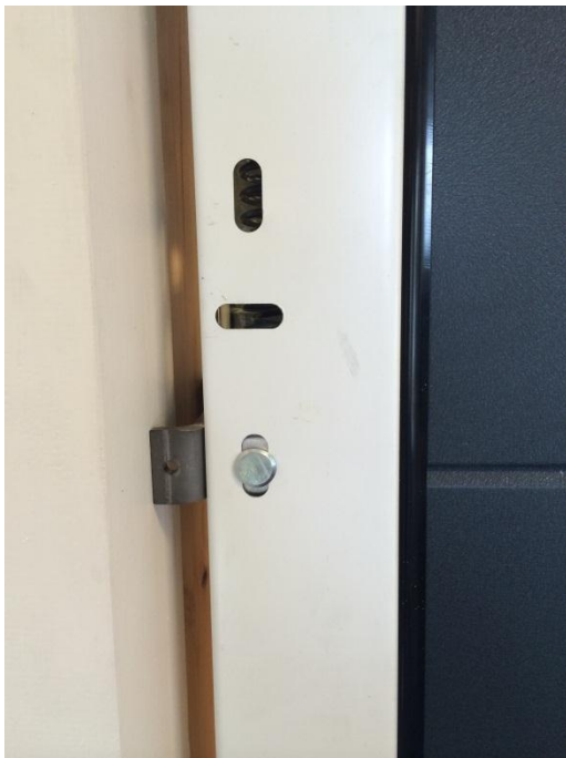
Fig 6 & 7 – Attach Cover Plate ( SG800C0 ) and rivet ( WI021WS ) to bracket, use touch up paint on rivets if required.
