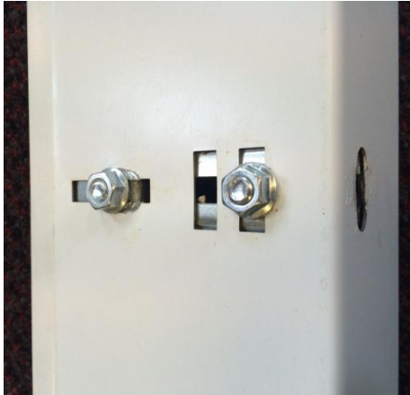
Fig 1 – Existing M8 x 15 Bolts & Nuts
