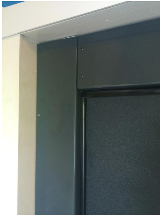
Fig 6 & 7 – Attach Cover Plate ( SG800C0 ) and rivet ( WI021WS ) to bracket, use touch up paint on rivets if required.
