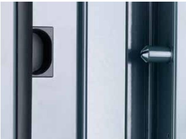
**Security bolts:** When the door is closed, they protrude into the frame and provide additional protection against forced entry.
